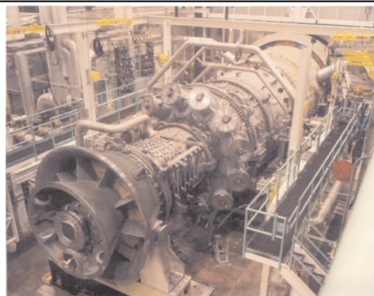
Figure 23. 7H gas turbine being installed in test stand
